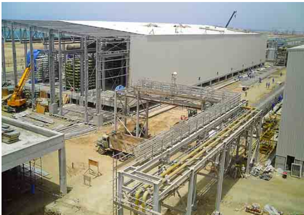
Power Generation and Water Desalination Facilities under Construction, Saudi Arabia
