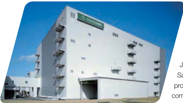
Pharmaceutical manufacturing plant for Dainippon Sumitomo Pharma Co., Ltd., Japan
