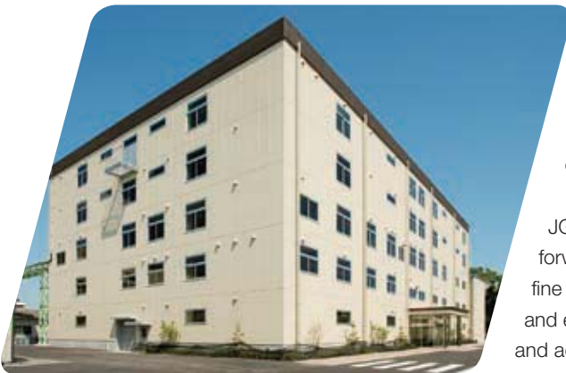
The new R&D center built by CCIC, Japan
