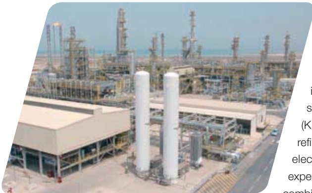
Petroleum refinery modernization project for BAPCO, Bahrain
