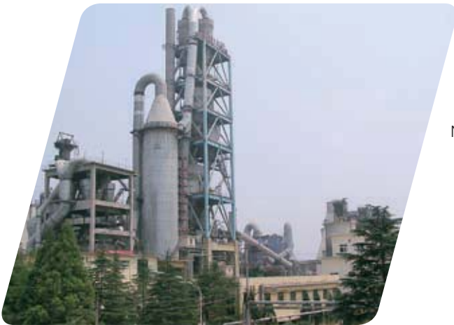
The Huaibei Cement Plant, promoting the CDM business with a waste-heat power generation facility, China
