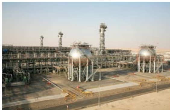
NGL recovery plant for Saudi Aramco, Saudi Arabia
