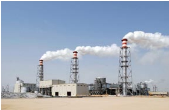
The Rabigh cogeneration, steam and desalination plant, Saudi Arabia
