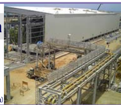
Water & Power facilities under construction (Saudi Arabia)
