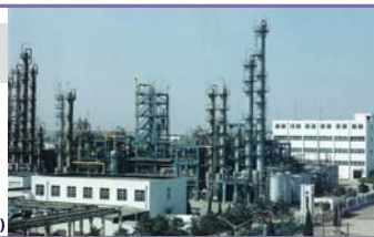
Juhua chemical plant (China)
