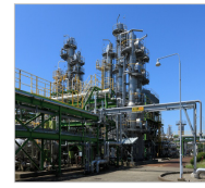
Testing new CO 2 recovery technology (INPEX Koshijihara Plant)
