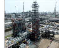
Demonstration facilities for propylene manufacturing technology
